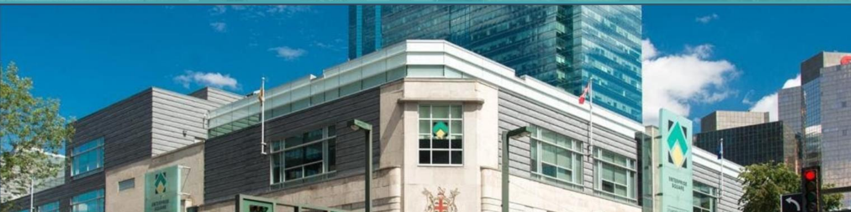
Head Office and HIH at Enterprise Square
